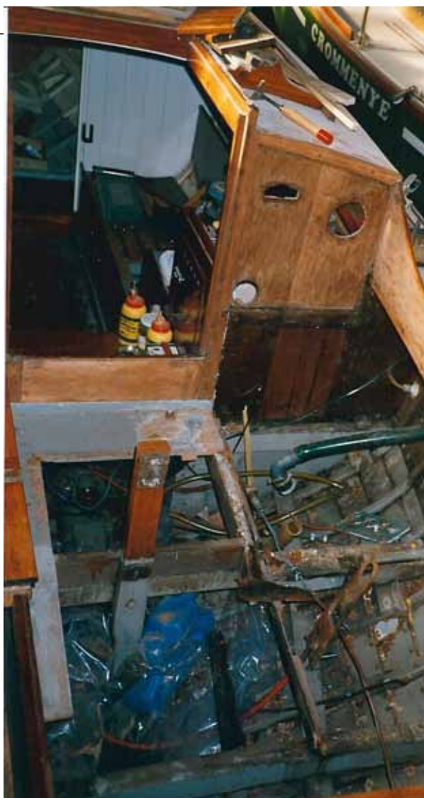
The cockpit rebuild on Scarlet
